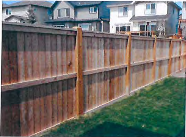
Figure 3-5 – Typical Neighborhood Fencing
